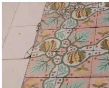
**Figure 11.** Detached, blunt, cracked and/or scratched tiles
