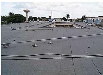
**Figure 4.** Asphalt blanket with granules
