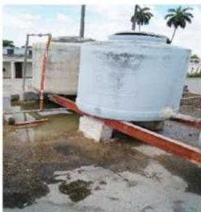
**Figure 10.** Overflow of water tanks
