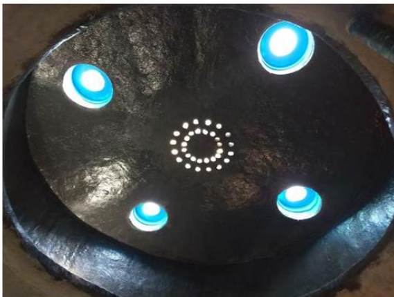
Figure 14 Application of FRP in the gas chamber (2022).
