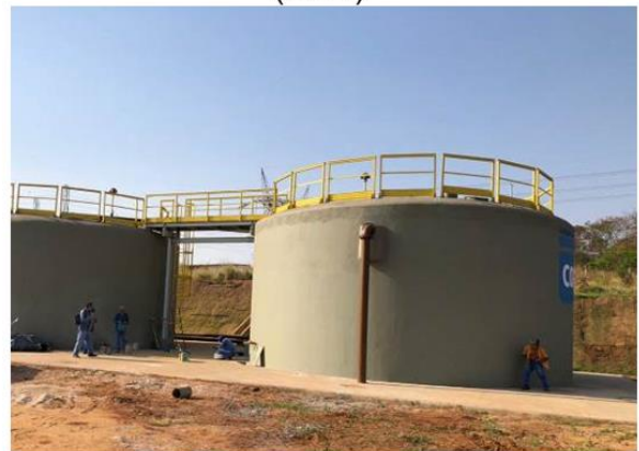
Figure 15 Installation of guardrails and access ladder to the reactor UASB (2022).
