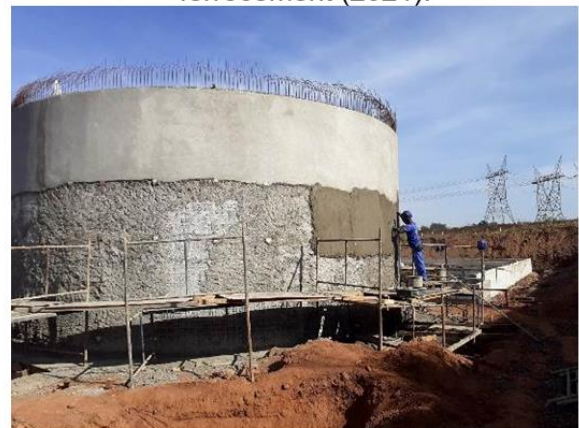
Figure 11 Application of the second layer of mortar on the external side of the wall (2021)
