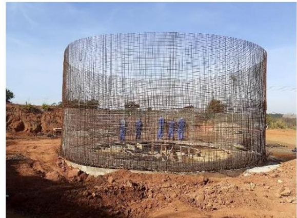
Figure 9 Execution of the reinforcement for ferrocement (2021).
