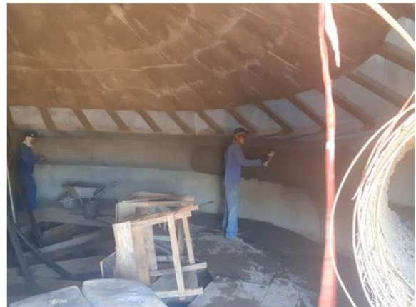
Figure 13 Working inside the reactor tank (2021).
