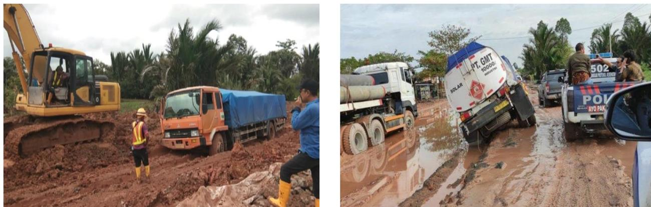
**Figure 1:** Lateritic soil as a subgrade road condition
