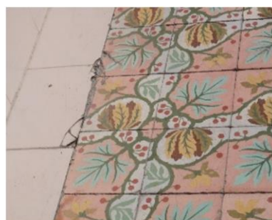
Figure 11. Detached, blunt, cracked and/or scratched tiles
