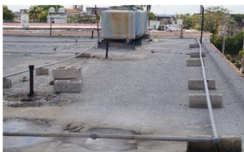
Figure 7. Distributor and elevated tanks
