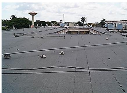
Figure 4. Asphalt blanket with granules
