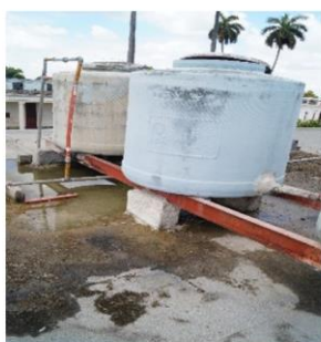
Figure 10. Overflow of water tanks
