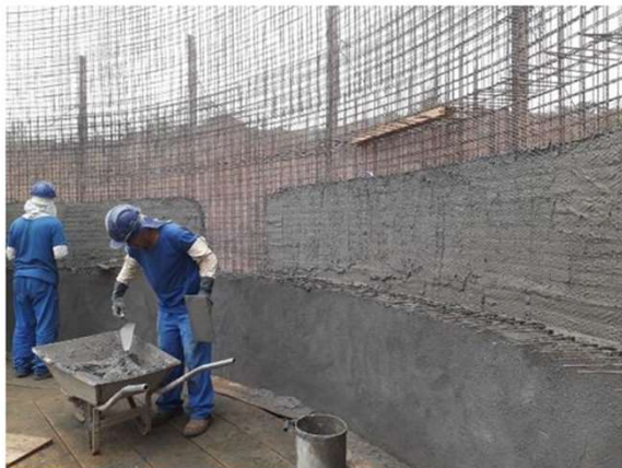
Figure 10 Application of mortar on the inner side of the wall (2021)
