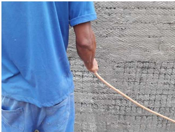
Figure 12 Cement curing water (2021)
