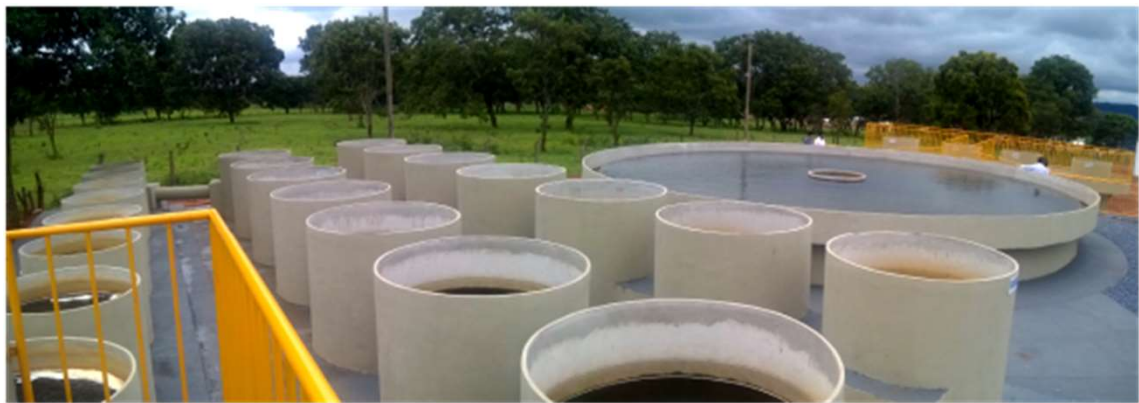
Figure 3 Water Treatment Plant in Ferrocement (flow = 24 L/S) Guimarães-MG, 2017.
