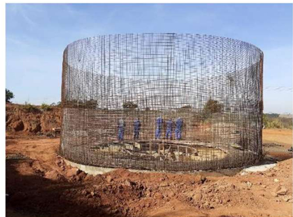
Figure 9 Execution of the reinforcement for ferrocement (2021).
