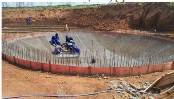
Figure 8 Execution of the reinforcement of bottom slab on ferrocement (2021).
