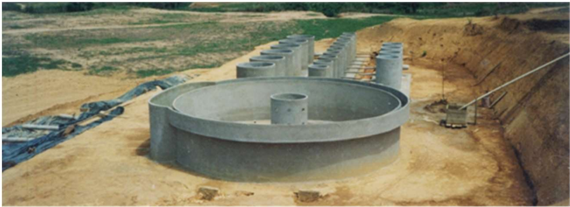
Figure 2 Water Treatment Plant in Ferrocement (flow = 12,0L/s) Pingo d'Água-MG, 1993.
